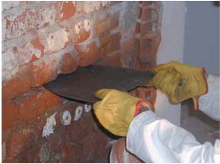
Figure 17: Flat jack being inserted into the slot
