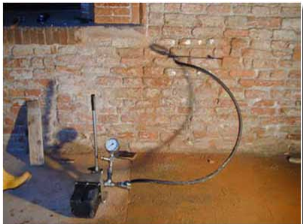
Figure 18: Equipment used to test stress
